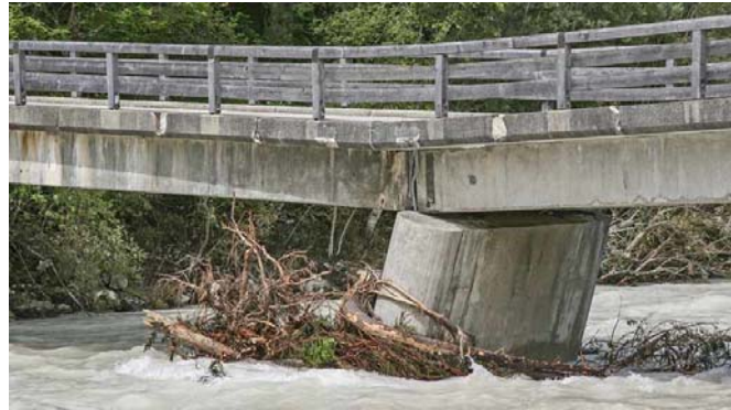
Figure 2. Accumulation of substantial amount of debris (trees, branches, leaves, sediment) on the upstream face of the pier. The debris piles up along the pier, reducing the flow profile. ( https://bridgemastersinc.com/protecting-bridges-flood-damage/ )
